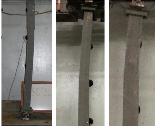
(a) Buckling of unreinforced segments
