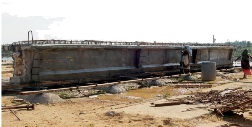
Fig. 2 Road bridge girder - after casting
