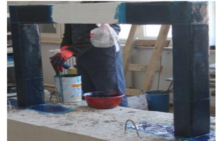
(f) Wrapping CFRP sheets with saturant material
