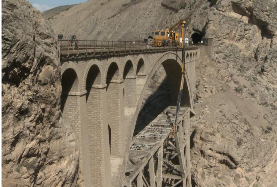
Fig. 5 Fixing DCDT's cable to the concrete structure beneath Veresk
