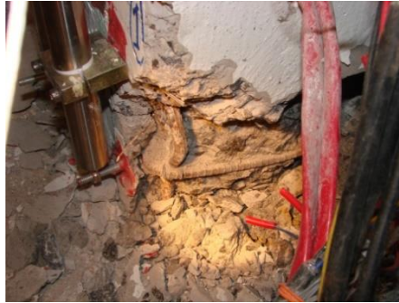
Fig. 7 Crushing of concrete in the compression zone and buckling of main bars
