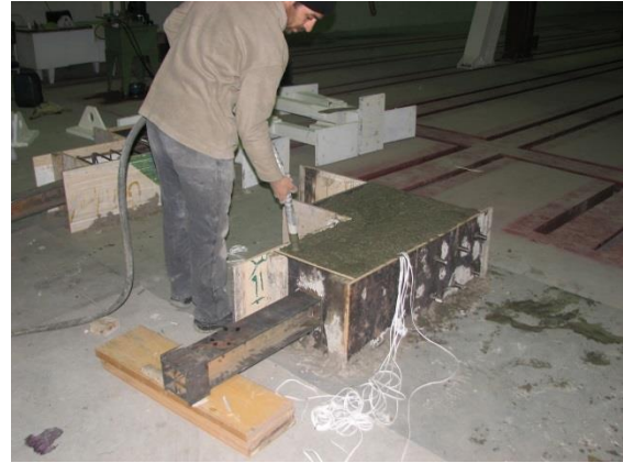
(b) Pouring of fresh concrete
