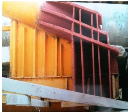
Fig. 12 Remedial Measure-II Implemented in real (i.e., as built) pipe-rack
