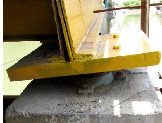
Fig. 2 A visible tilt in the bearing plate
