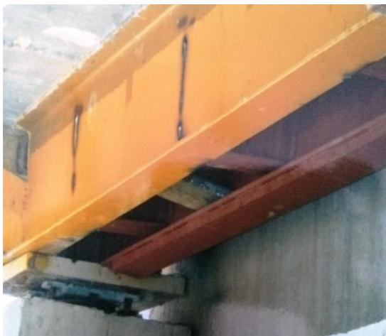
Fig. 11 Remedial Measure-I Implemented in real (i.e., as built) pipe-rack
