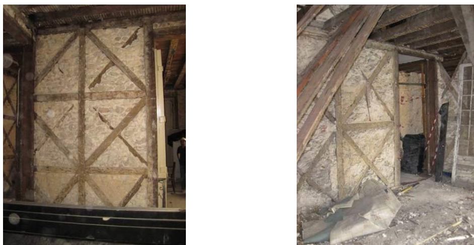
Fig. 1 Timber framed wall in “pombalino” building (Gonçalves et al. 2011)
