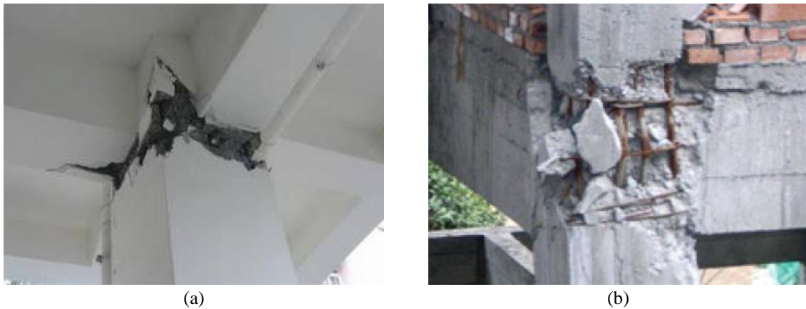
Fig. 2 Beam-column joints damaged during the China Wenchuan earthquake of May 12 2008
