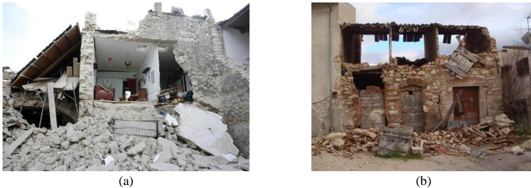
Fig. 1 Out-of-plane collapse of unreinforced masonry facade walls after the 2009 L'Áquila earthquake: (a) global overturning and (b) partial collapse
