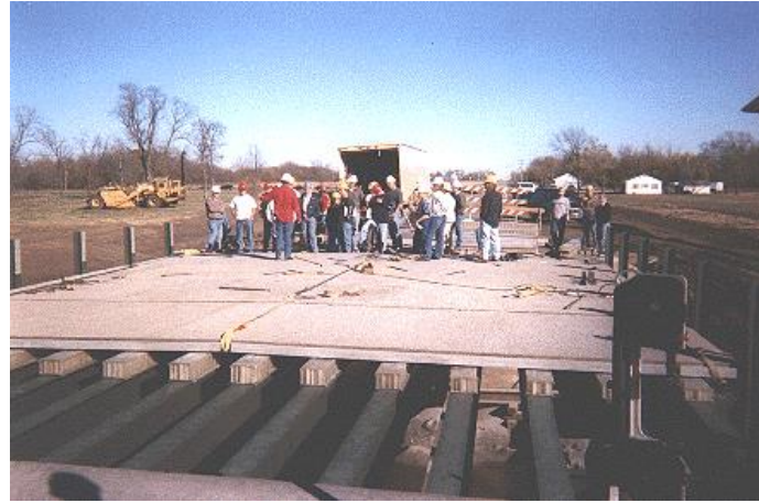
Fig. 1 GFRP honeycomb hollow section sandwich panel bridge, KS
