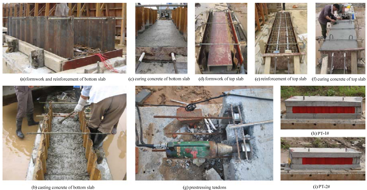
Fig. 2 Fabrication of a composite box girder with corrugated steel webs
