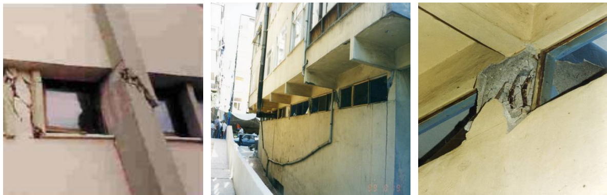
Fig. 1 Short column damages
