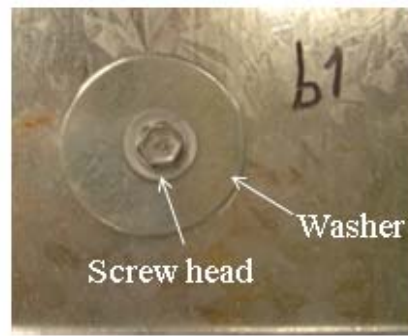
Fig. 5 Details of washer and improved connection
