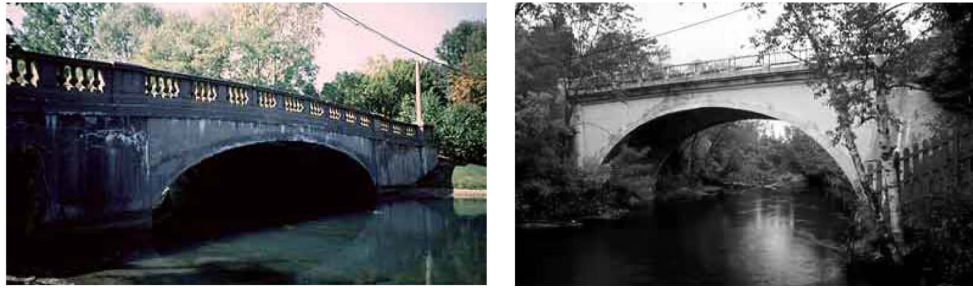
Fig. 1 Typical single span reinforced concrete historic bridges with symmetrical parabolic haunches having the constant haunch length ratio of 0.5
