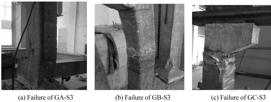
Fig. 9 Failure patterns of columns with e/t = 0.50
