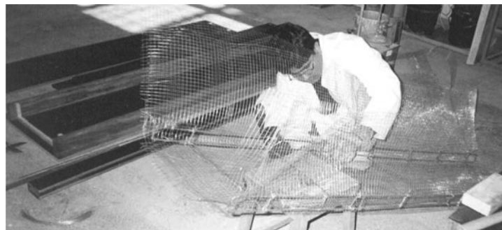
Fig. 16 Method of construction of a typical panel
