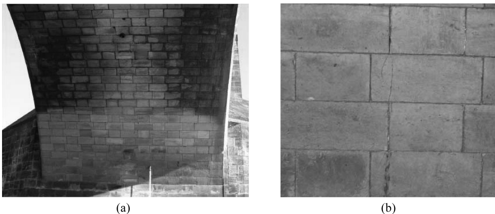
Fig. 1 (a) A view of a typical bridge arch showing a regular arrangement of stones in masonry, (b) a crack running both across stone and along a head joint
