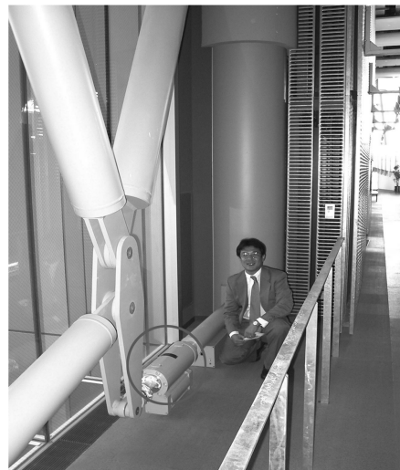
(b) Installation of an MR fluid damper
