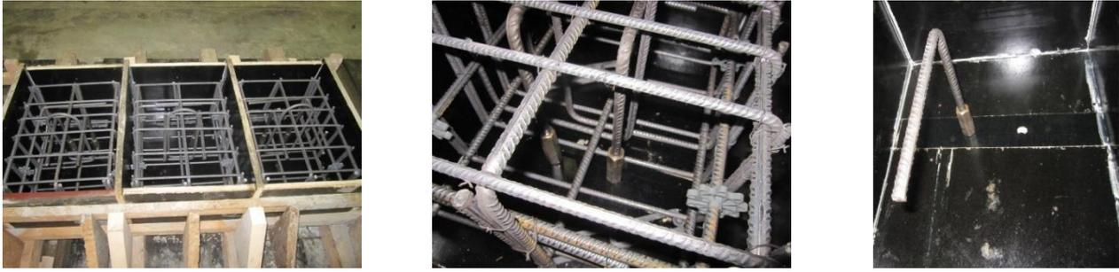
Fig. 3 Shear connector's attachment to the formwork
