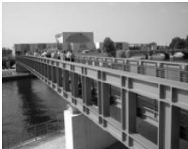
Fig. 4 Vierendeel frame used in the construction of a bridge
