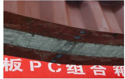
(f) Cracks on bottom slab
