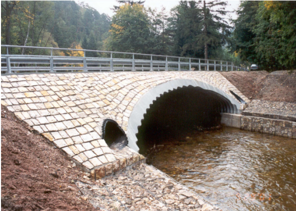
Fig. 1 Side view on the analyzed SSC culvert
