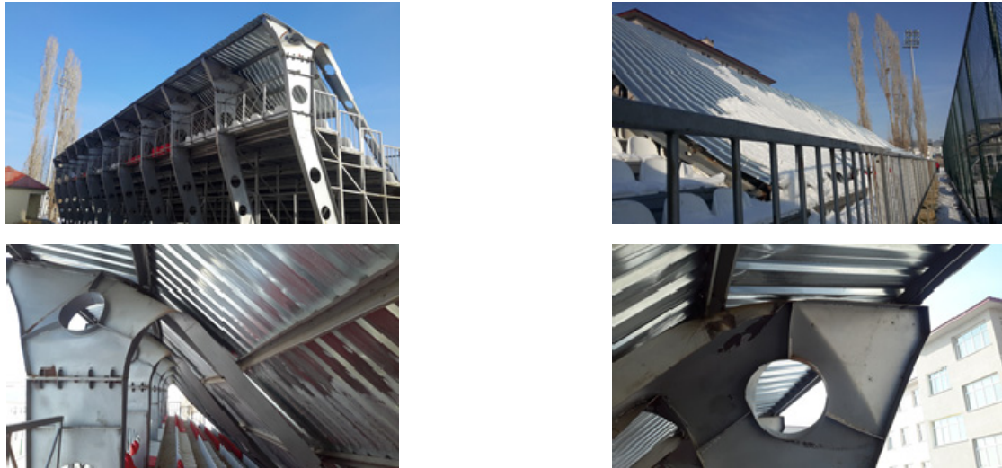
Fig. 3 Some views of completely collapsed cantilever roof of tribune structure
