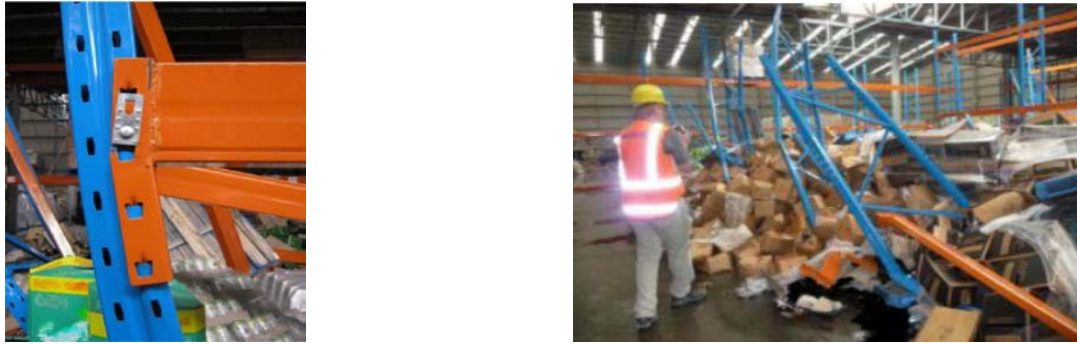
Fig. 2 Collapsed rack system in Christchurch earthquake in 2011 (Clifton et al. 2011)
