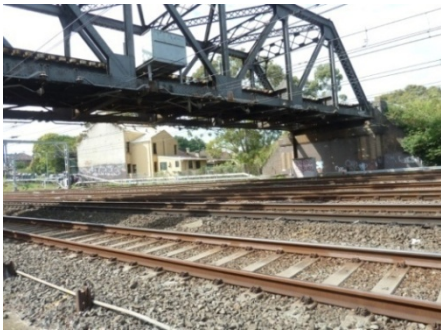
(a) Typical elevated transom bridge with vertical space constraints from roof trusses
