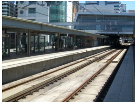
(c) Railway slab track or direct fixation adjacent to existing platforms
