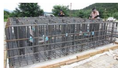
(c) Rebar arrangement of footing
