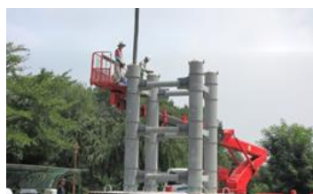
(b) CFT tube assembly
