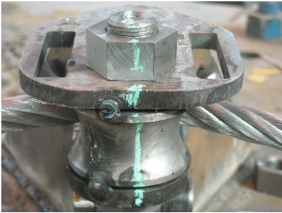
Fig. 8 Rolling cable-strut joint
