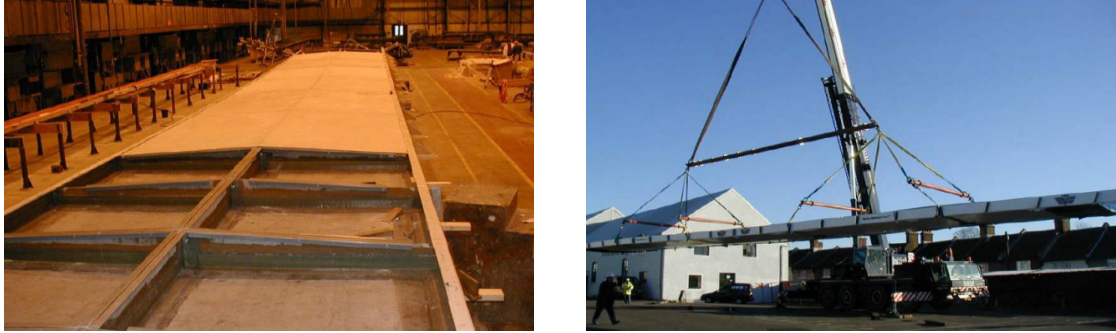
Fig. 2 Bridge deck of Halgavor suspension footbridge (URL 2012a)
