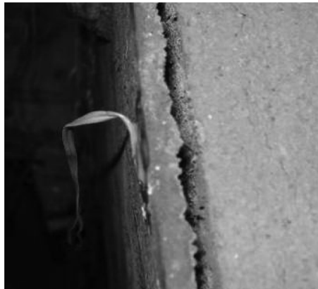
Fig. 7 Separation between steel plate and masonry
