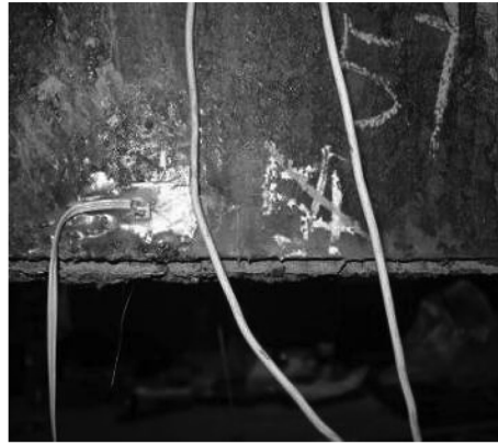
Fig. 9 Encased masonry gliding downward
