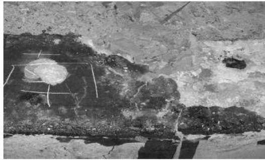
Fig. 11 Masonry crushing in compression zone
