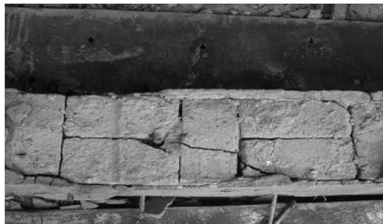
Fig. 10 Damaged masonry of beam L1
