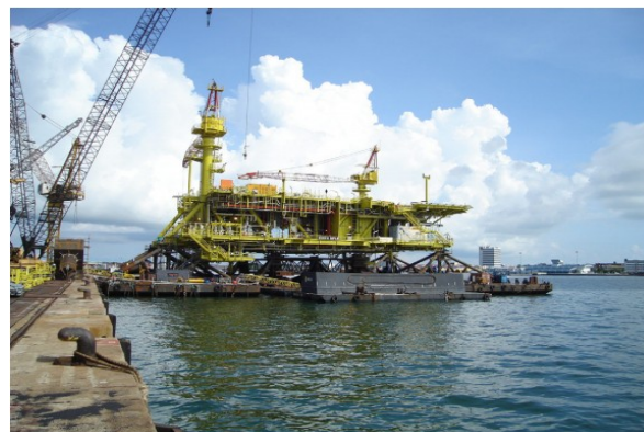
Fig. 1 Transport barge and floatover barges in position
