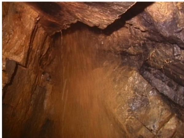
Fig. 18 Water inrush occurred in karst conduit (PDK354+235)
