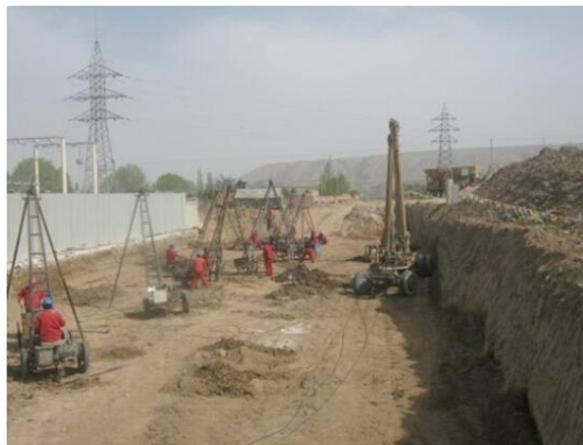
Fig. 5 The holing construction of compaction piles
