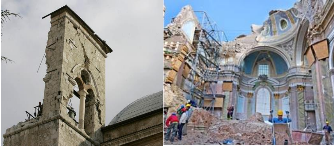
Fig. 4 Observed damage on URM buildings due to intraplate earthquakes after the M6.3 L'Aquila, Italy earthquake occurred in 2009
