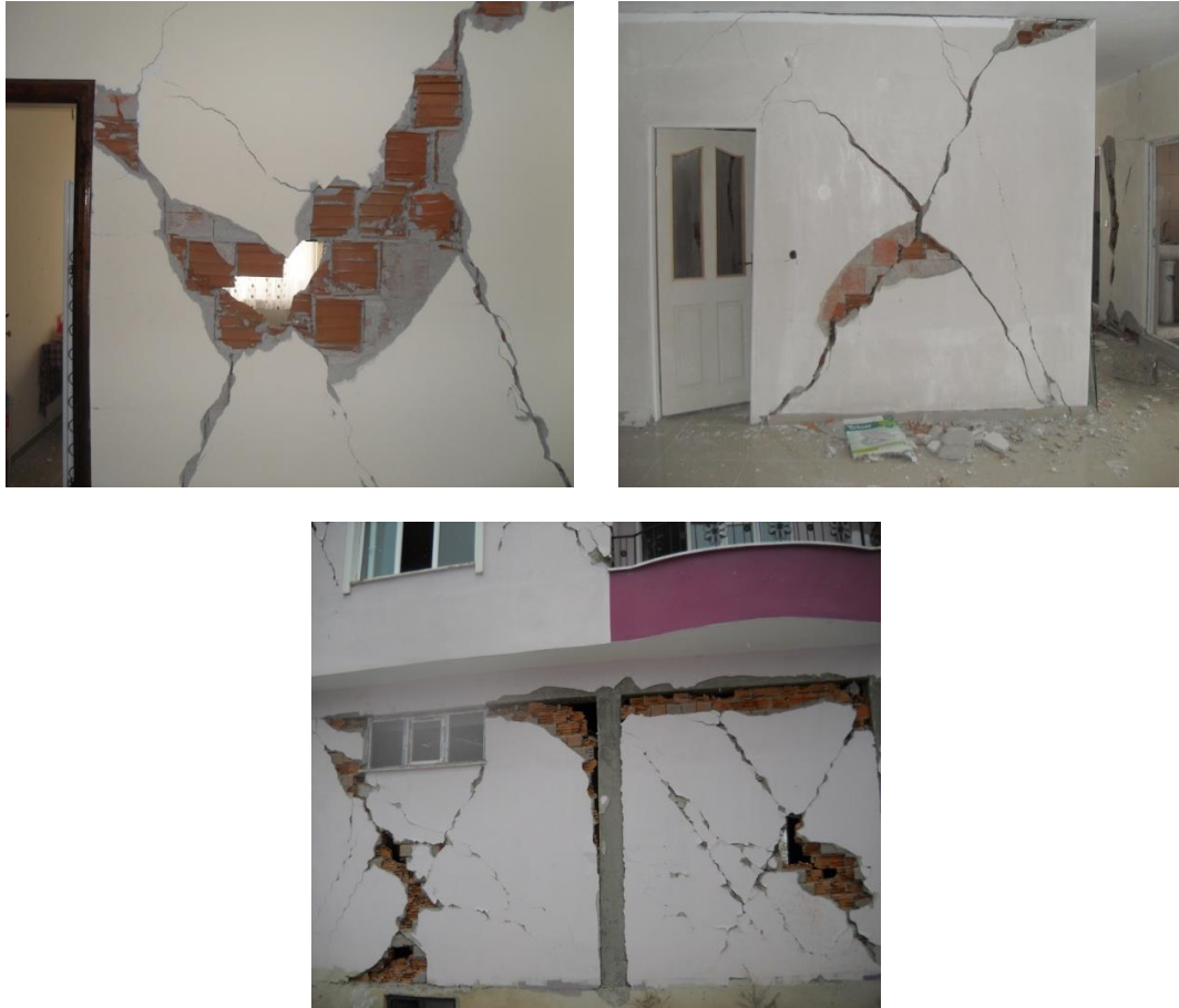
Fig. 23 In plane failure mechanism in infill walls at some R/C buildings
