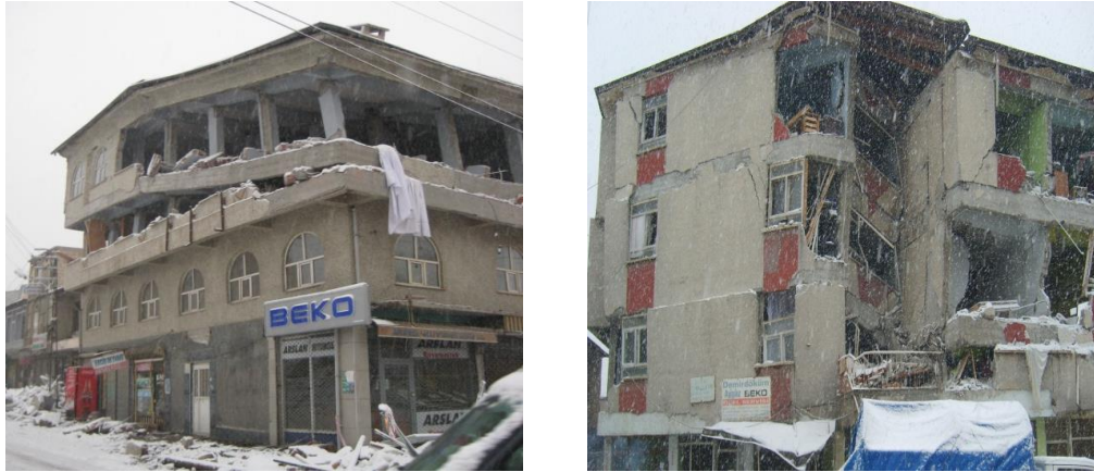
Fig. 13 Weak storey mechanism at various R/C buildings
