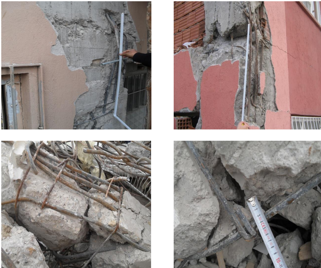
Fig. 14 Inadequate transverse reinforcement, improper hooks and smooth bars
