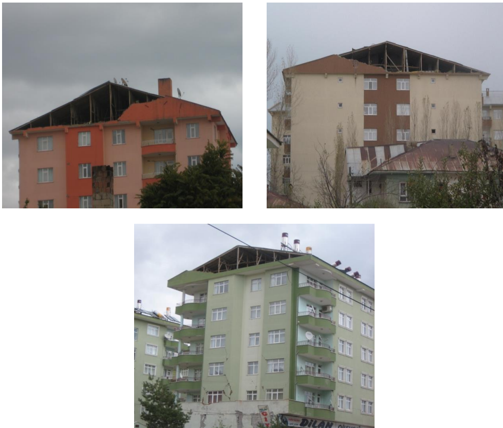
Fig. 19 Out-of-plane failures of gable walls at various buildings
