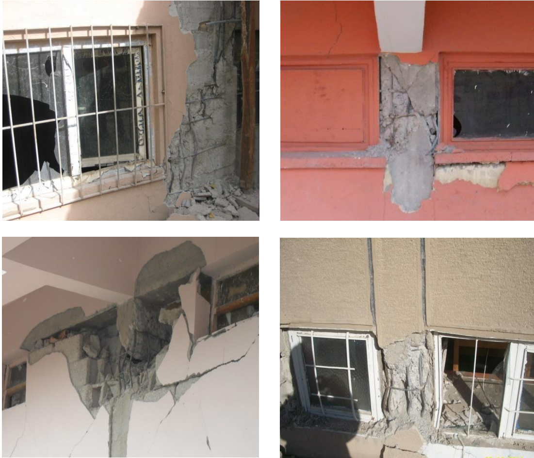
Fig.16 Short column damages at various buildings
