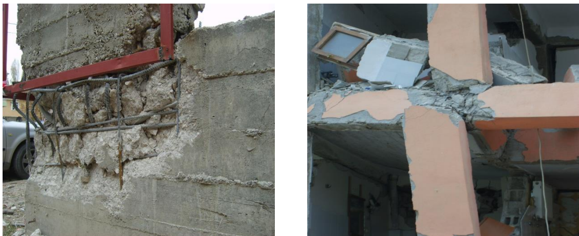
Fig. 15 Joint failures at various reinforced concrete buildings
