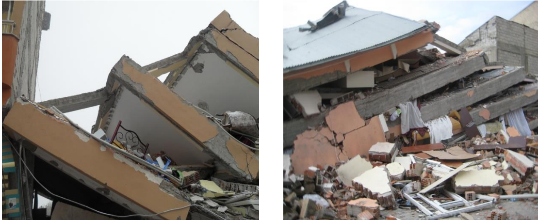
Fig. 18 Total collapses at various buildings due to strong beam-weak column
