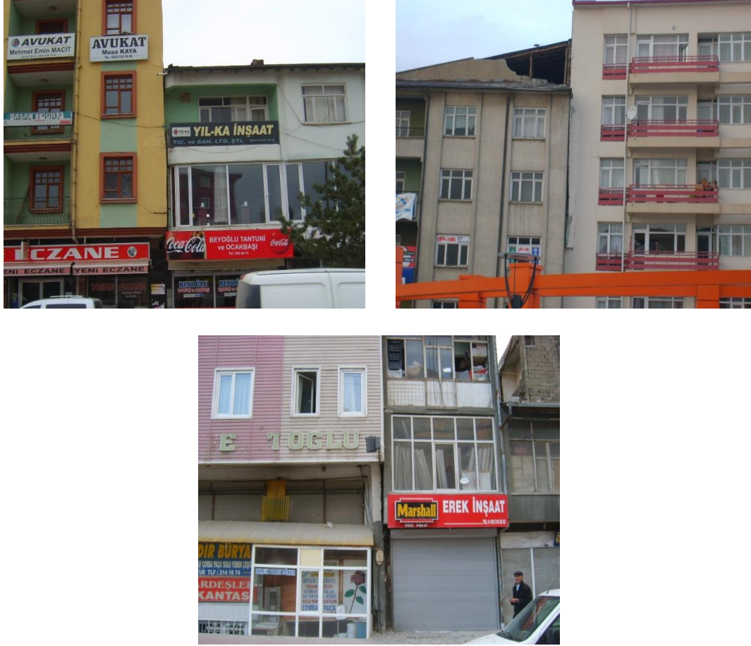
Fig. 17 Inadequate gap between adjacent buildings and damages
