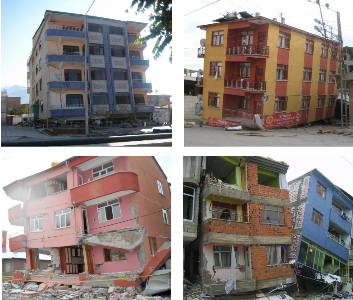
Fig. 11 Soft storey mechanism at various reinforced concrete buildings
