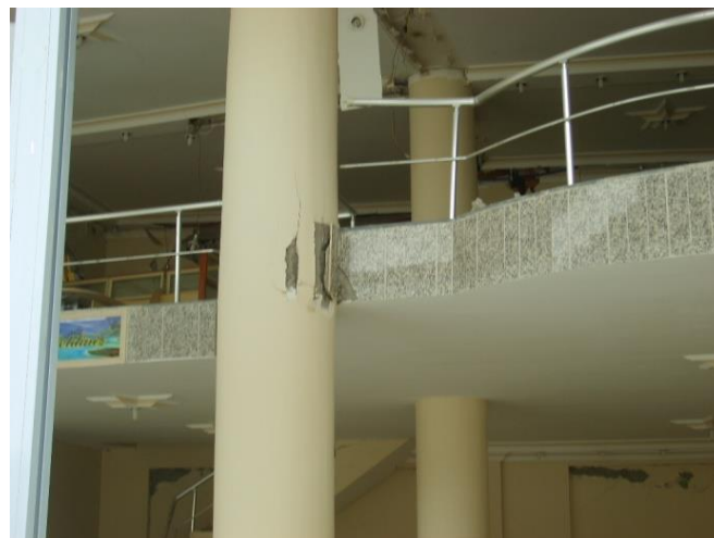
Fig. 12 Damage at a column due to mezzanine
