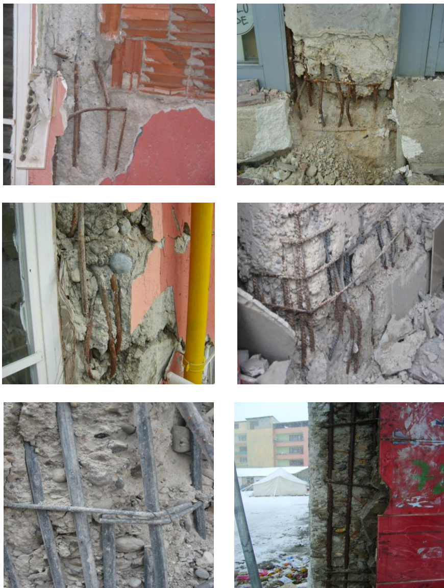
Fig. 21 Corrosion, smooth reinforcement and improper granulometry at columns of different buildings
