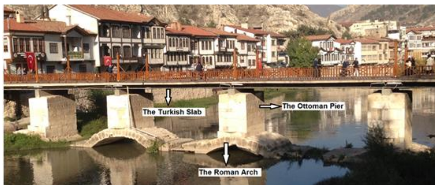
Fig. 4 Structural components of the bridge
