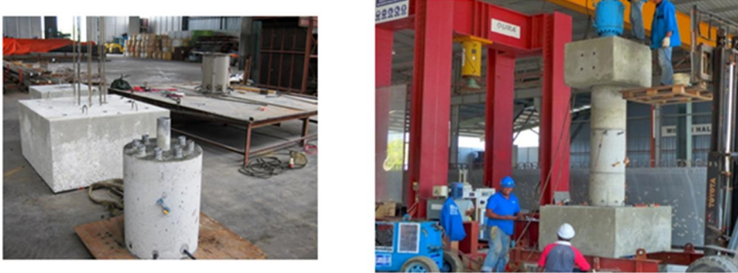
Fig. 3 Precast footing, load stub and the segments of the specimen before and after assembling
