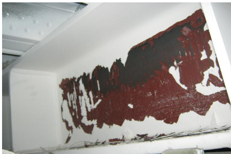
Fig. 10 Active link beam from Club Tower, Christchurch which has undergone plastic strain
