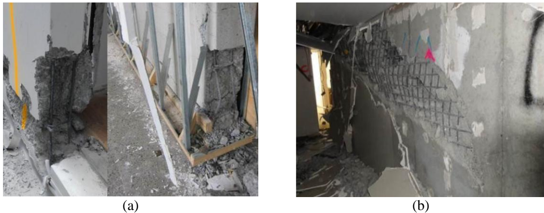
Fig. 2 (a) Bar buckling and fracture in lightly reinforced slender RC shear wall; (b) Slender wall shear-axial failure (Kam et al. 2011)
