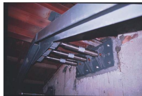
Fig. 13 Shape memory alloy device insertion for the San Feliciano Cathedral façade (Indirli and Castellano 2008)
