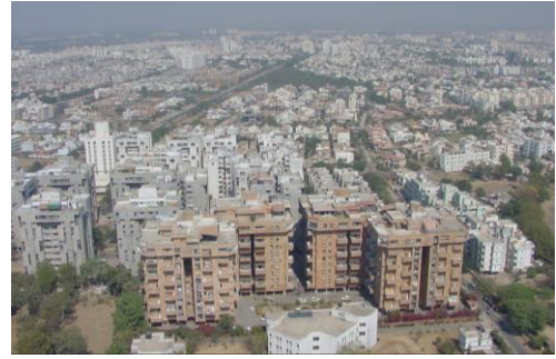
Fig. 3 Typical skyline of cities showing reinforced concrete (RC) frame buildings with extreme stiffness irregularity due to open storey at ground level
