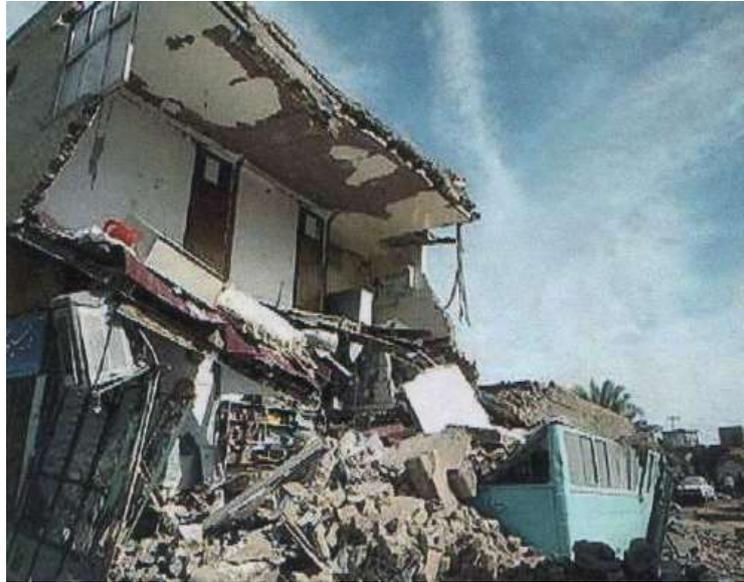
Fig. 1 Out-of-plane failure of URM walls (Kanit and Atimtay 2006)
