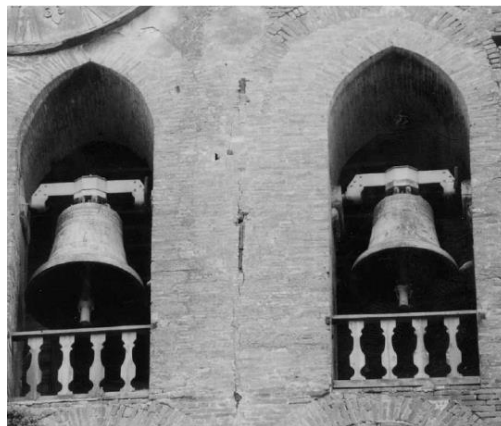
(a) Location of bells at belfry and crack pattern
