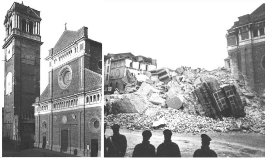
Fig. 7 The collapse of the historical civic tower of Pavia in 1989 (Binda 2008)
