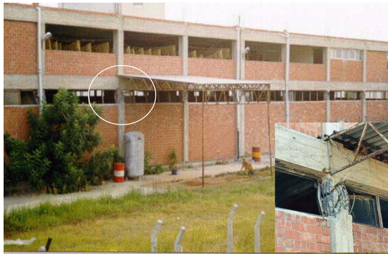
Fig. 9 Overview of the case-study building
