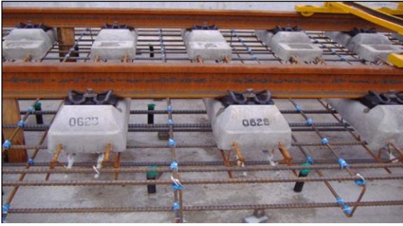
Fig. 1 Steel reinforcements in the concrete slab track system
