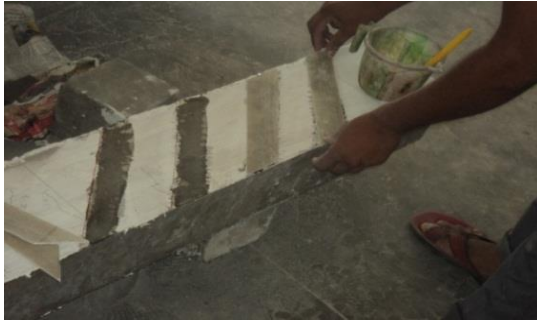
Fig. 6 Bonding of GFRP
