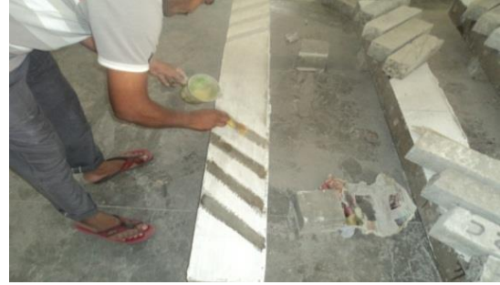
Fig. 5 Epoxy coating
