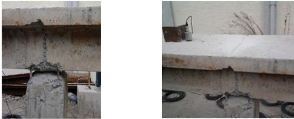
b) Cracks along to the lateral direction on bridge deck
