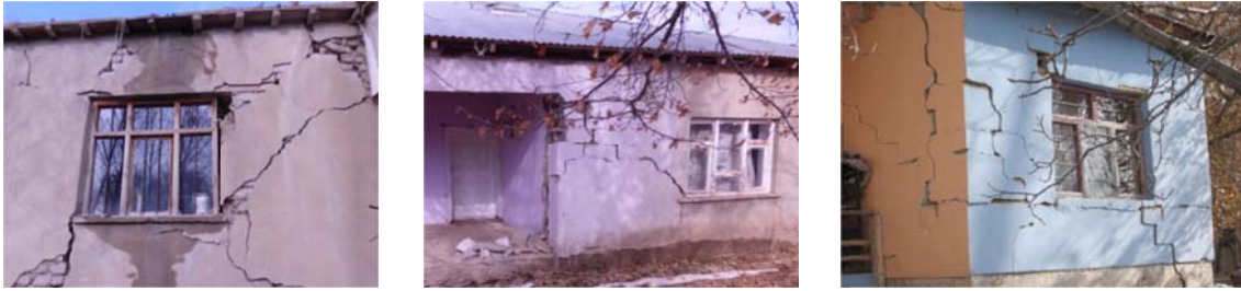
Fig. 1 Failure modes of masonry walls with an opening
