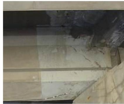
(b) Typical mortar repair of girder end
