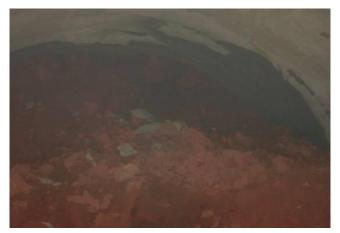
Fig. 8 Collapse body upper right's fissure water in right tunnel
