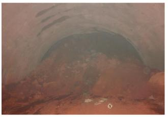
Fig. 7 Collapse situation of the right tunnel
